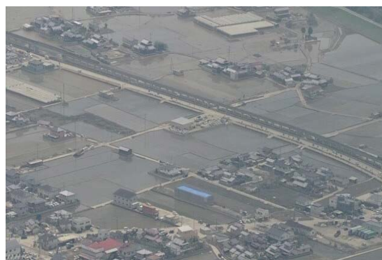
Fig. 1 Photograph of flood damage site caused by the extremely heavy rain in western Japan region in Mabi-cho, Kurashiki-shi, Okayama Prefecture 1)
